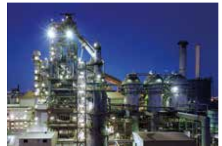
For use in petrochemical and iron & steel industries
