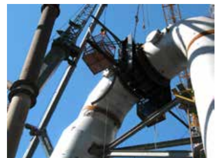
Site installation of an open type Goggle Valve
